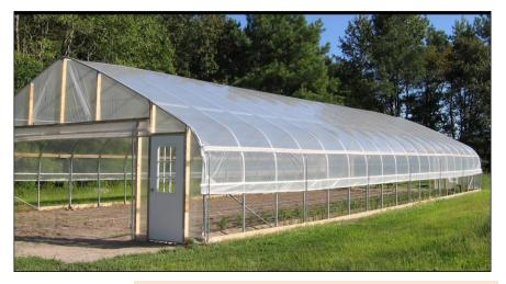
A <u>high tunnel</u>, which is sometimes called a hoop house, is a metal framed structure covered with greenhouse plastic. They look a lot like a greenhouse, but they generally don't have an artificial heating source, and plants are grown in the ground as opposed to in pots.
